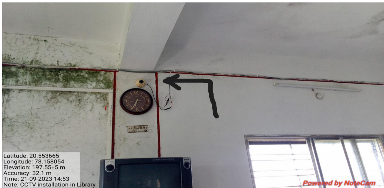
CCTV CAMERA INSTALLATION IN LIBRARY
